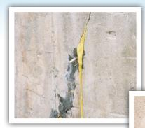
Optional polyurethane injection stops water from the outside of the wall (for really severe leaks).
