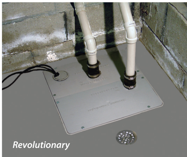
Water Grabber® Bull Dog™ with two pumps and top discharge.
